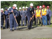
Eighteen months ago Jeff Pitzer drove a shovel into a large patch of dirt to ceremoniously break ground in what is now the new Storehouse and Maintenance Shops Complex.
